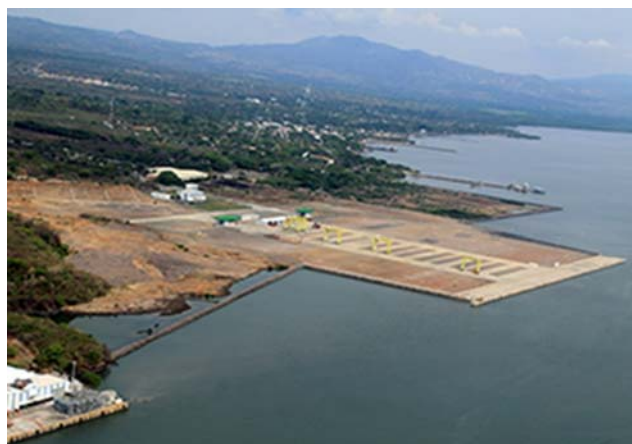
Puerto La Union Wharf from SE
