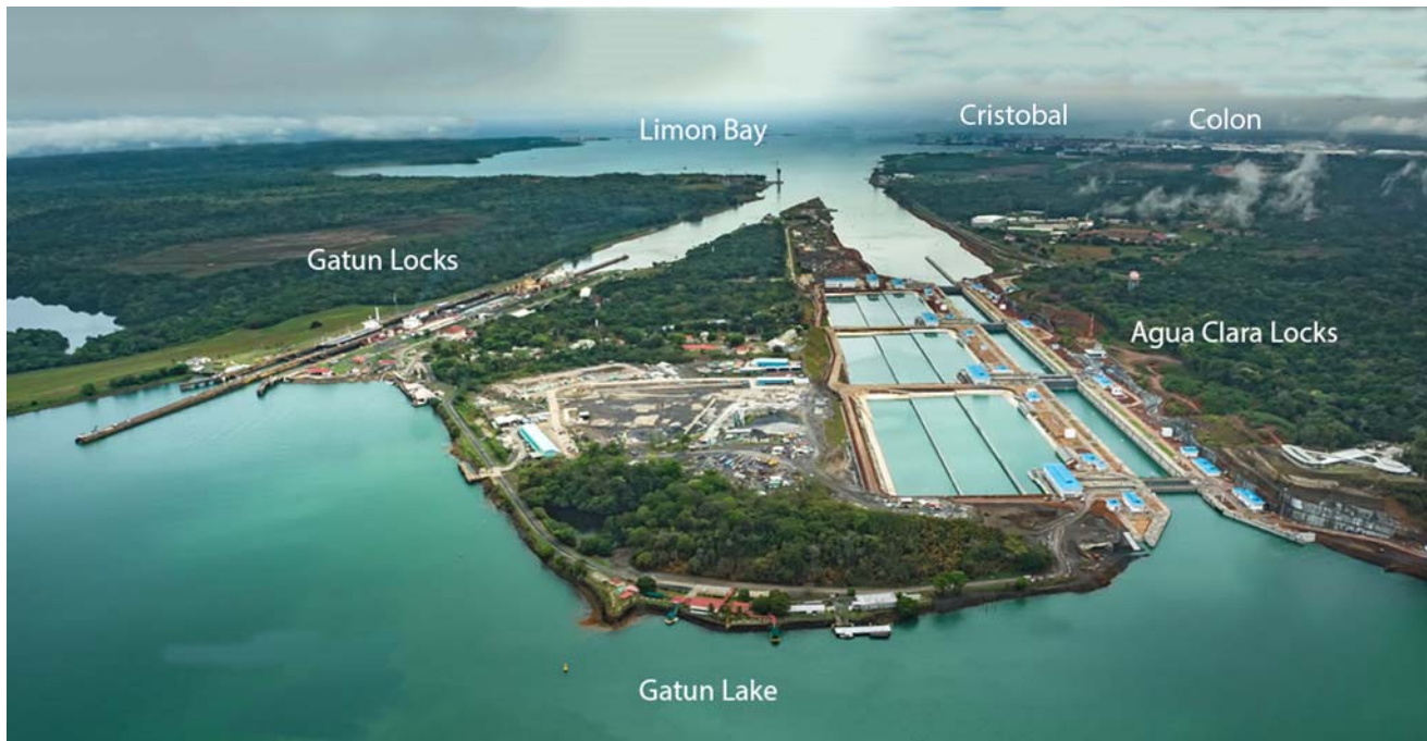
Agua Clara Locks Outbound (Neopanamax/Atlantic side)—Gatun Lock on the left side
