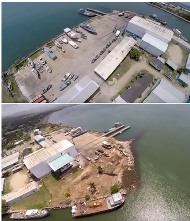
Puerto Cortes Naval Port Piers W of Isla Santa Margarita
