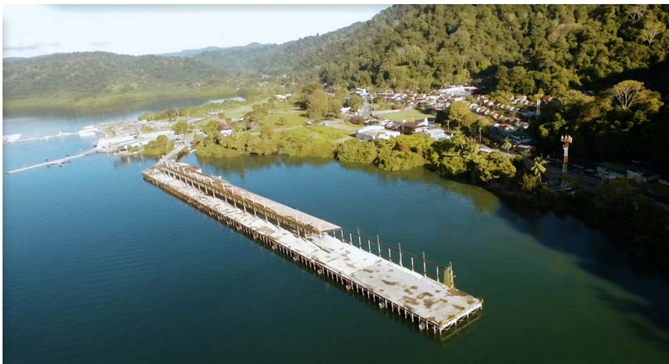
Golfito Main Wharf
